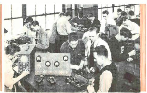
Here you see an Instructor giving students in our Industrial Electronics Department special instruction in checking the characteristics of high vacuum type tubes, using a specially constructed testing unit.
