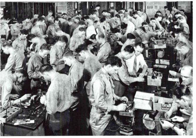
This photo shows a section of the Radio Servicing Department at Coyne. Here students learn to do layout of chassis, build and wire Receivers and do Trouble Shooting and Testing. Plenty of Sets, Parts, Instruments and tools are provided to make the training intensely practical. Experienced instructors help students with their Shop Work and answer their questions.
