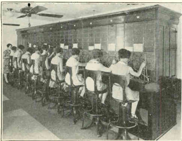
Fig. 147-F. This photograph shows a section of a large manual telephone exchange. Each operator controls a section of the board with its respective plugs and jacks.
