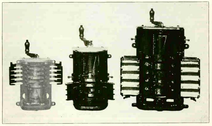
Fig. 143. The above photo shows several types and sizes of modern drum controllers. Examine arrangement of parts of each of these controls.
