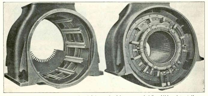
Fig. 85. The above two views show very clearly the method of construction of the stator core and windings of high speed steam-turbinedriven alternators.
