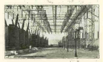
Fig. 414. View of large oil switches and lightning a resters underneath the bus and switching structure of a 220,000-volt outdoor substation. (Courtesy of Philadelphia Electric Company.)
