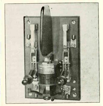
Fig. 420. Small air circuit-breaker for use on circuits of 600-volts and loads up to 400 amperes. Note the flash barrier placed between the two poles of the breaker. (Courtesy of G. E. Company.)
