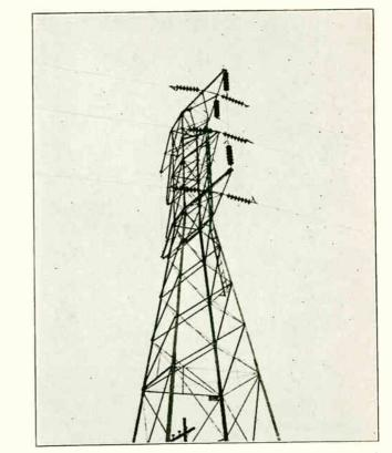
Fig. 356. The above photo shows a transposition tower in a highvoltage line. Note carefully the arrangement of insulators and conductors, and compare this photo with the lower sketch in Fig. 355.
