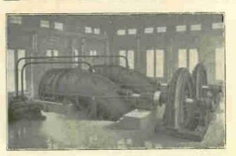
Fig. 195. This photo shows 2600-h. p. synchronous motors driving lowpressure, screw type water pumps. (Photo courtesy Allis-Chalmers Mfg. Co.)
