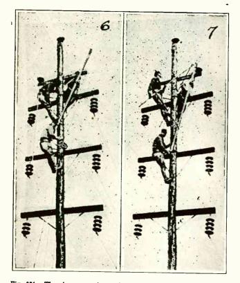
Fig. 371. The above two photos show linemen at work on a "hot" or live line, replacing insulators by means of live line tools. This work requires extreme care and accuracy and is generally done by specially trained line crews. (Courtesy Johnson Mfg. Co.)
