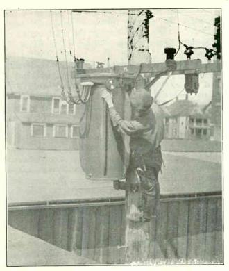
Fig. 124. This photo shows a pole type transformer and the method of making primary and secondary connections. Also note the thermotel temperature indicator near the hand of the electrician.
