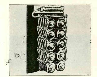
Fig. 234. Copper oxide rectifier consisting of a number of units connected in series and parallel to obtain increased voltage and current capacity. (Courtesy Westinghouse Elec. & Mfg. Co.)
