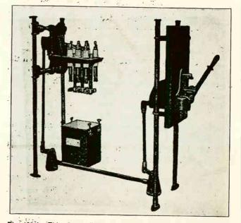
Fig. 422-A. This figure illustrates the method of obtaining remote mechanical control for an oil switch located several feet back of the switchboard. (Courtesy of G. E. Company.)
