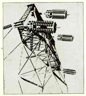
Fig. 346. Extra heavy strain tower with six strings of insulators grouped together on evener plates for each conductor. Note the heavy coll springs on the left evener plates to allow the heavy tension of these 3800-ft. river spans to equalize on all six insulator strings. (Courtesy Lapp Insulator Co., Inc.)
