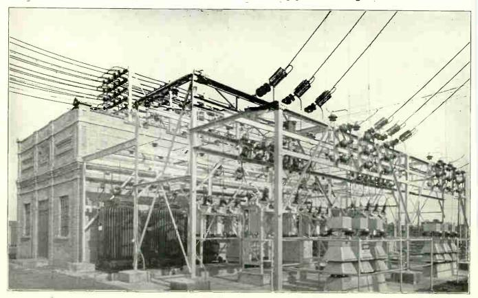
Fig. 388. This photo shows an excellent view of a substation with two sets of three-phase lightning arresters in the foreground, and their choke coils and disconnect switches directly above them. Also note the oil switches and step-down transformers in the background. (Courtey G. E. Company.)
