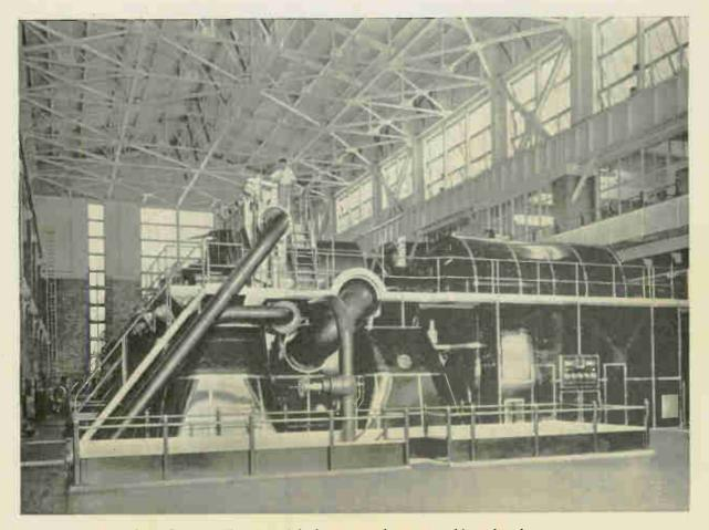
A modern General Electric vertical-compound steam turbine electric generator set, 110,000 K.W. This unit has hydrogen-cooled generators and includes the most modern improvements in large generating equipment.
