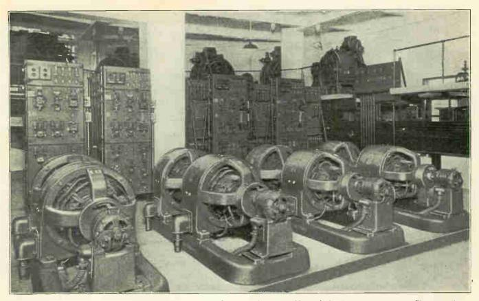
Fig. 132-C. This view shows the control panels for a group of modern elevator machines of the motor-generator type. The magnetic contactors on these panels are operated by remote control from the elevator car.
