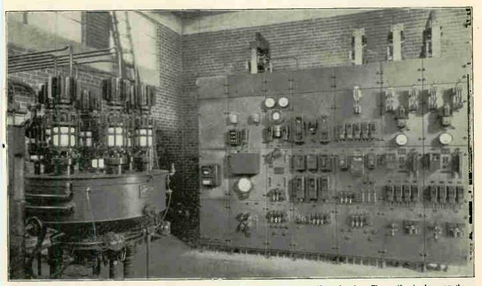
Fig. 411. This photo shows an excellent view of the interior of an automatic mercury arc rectifier substation. The rectifier is shown on the left and the automatic control switchboard with its relays and circuit breakers is shown on the right. (Courtesy of General Electric Co.)
