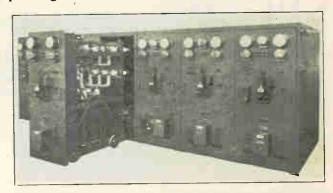
Fig. 418. View of truck-type switchboard showing one section removed to allow repairs or adjustments to be conveniently and safely made. Boards of this type are very popular in modern industrial plants as well as in certain power plants and substations. (Courtesy of G. E. Company.)
