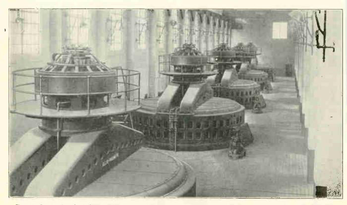
Fig. 317. Interior view of a bydro-electric generating station showing a row of large water-wheel-driven vertical type alternators. The water wheels are located beneath the generator floor and direct-connected to the vertical shafts of the generators. Each unit develops 17,500 horsepower at 100 RPM. (Courtesy Allis-Chalmers Mfg. Co.)
