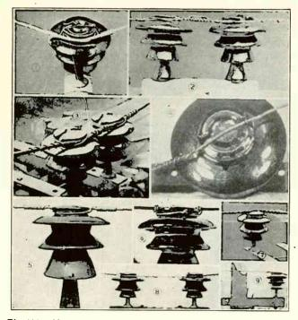
Fig. 334. Above are shown a number of common types of line ties used for attaching conductors of transmission and distribution lines to pin type insulators. Examine each type very carefully as you read the accompanying descriptions and also compare them with the sketches in Fig. 335. (Courtesy Lapp Insulator Company, Inc.)
