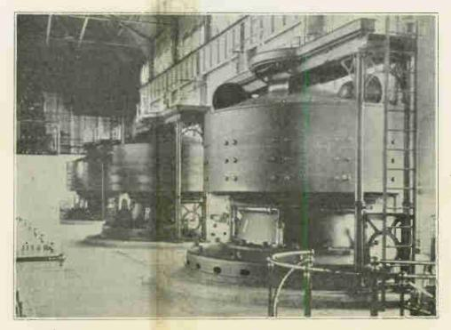
First Alternating-Current Generators installed at Niagara Falls in 1895 by Westinghouse Electric & Manufacturing Co.
