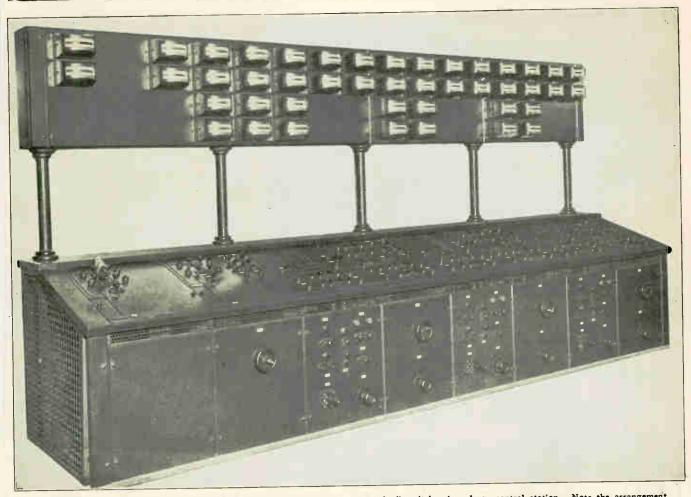
Fig. 417. Modern bench-type switchboard for remote control of genera ors and oil switches in a large central station. Note the arrangement of the meters and the push-pull switches which control the solenoid operated and motor-operated oil switches and devices throughout the plant. (Courtesy of G. E. Company.)
