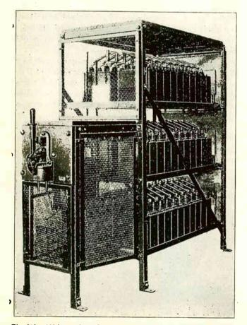
Fig. 213. 300-kv-a., three-phase, 2500-volt, capacitor or static condenser, used for improving power factor. (Courtesy General Electric Co.)
