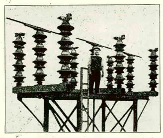
Fig. 434. Three-pole air break switch for use on 154,000-volt, threephase lines. Note the rotating blades which are abown in open position in this view. (Courtesy of Delta-Star Mfg. Co.)
