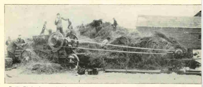
Fig. 211. This photo shows a portable A. C. motor driving a hay baler. Many thousands of farms are making excellent use of electricity to save time and money in many ways, and taking advantage of the increased safety obtained by use of electrical power equipment. (Photo courtesy G. E. Company)
