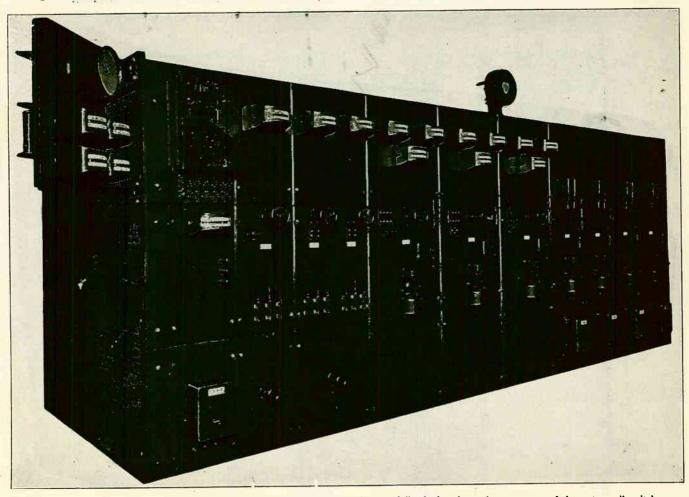
Fig. 415. An excellent view of a modern panel-type A. C. switchboard. Note carefully the location and arrangement of the meters, oil switches, (Courtesy of G. E. Company.)
