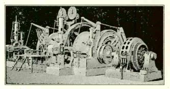
Fig. 187. Large slip-ring motor used to drive the drums of a hoisting machine. Note the manner in which the stator leads are brought up to the motor in conduit which is imbedded in the floor. (Photo courtesy Allis-Chalmers Mfg. Co.)
