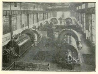
Fig. 304. Interior view of a large power plant showing several modern steam turbine-driven alternators.
