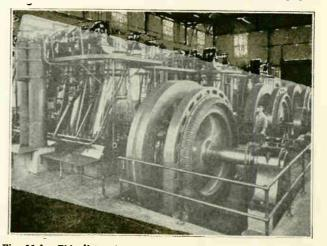
Fig. 95-A. This photo shows a group of alternators driven by Diesel oil engines. Many power plants located in the oil fields, or in places where water and coal are difficult to obtain, are equipped engines and generators of this type.
