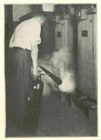
Fig. 474. This photo ahows the use of a modern gas type fire extinguisher for fire protection in electric plants.
