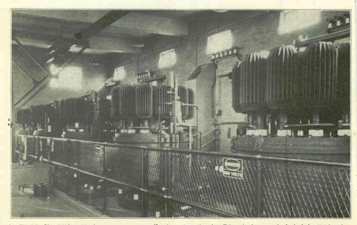
Fig. 248. Five 1200-kw., 600-volt, mercury arc power rectifiers in use in a sub-station. This station has a capacity for producing 6000 kw. of rectified D. C. from the alternating current supplied. / (Photo courtesy American Brown Boveri Co.).
