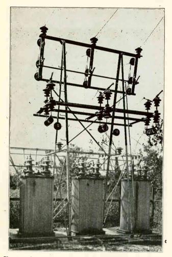
Fig. 401. Small outdoor transformer substation with transformers located on a base on the ground, and chock coils, fuses, and disconnect switches on the steel tower above them.
