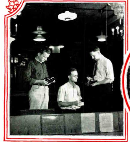
These students are making practical tests on various lighting fixtures with foot-candle meters and light meters. Their instructor is giving them a personal explanation of one of the modern type photocell foot-candle meters.
