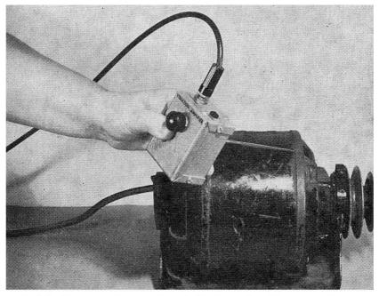
Fig. 7-8.—Using a transistorized electronic "Stethoscope" to listen to the vibration of an electric motor.
