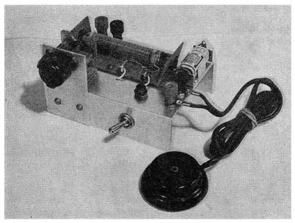
Fig. 8-2.-Overall view of the Simple Receiver.
