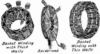
Fig. 3.—Types of Coils Showing Various Resistances.
