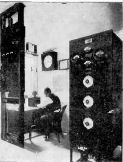
Fig. 3. Main control panels of a Radio Broadcast Station.
