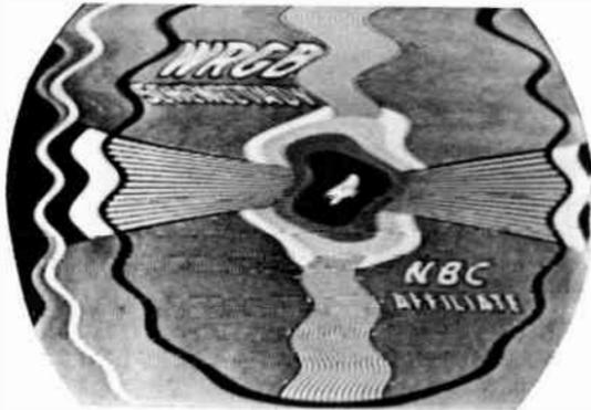
Fig. 1-P. *Pie-crust effect in pix.* courtesy G-E Techni-talk
