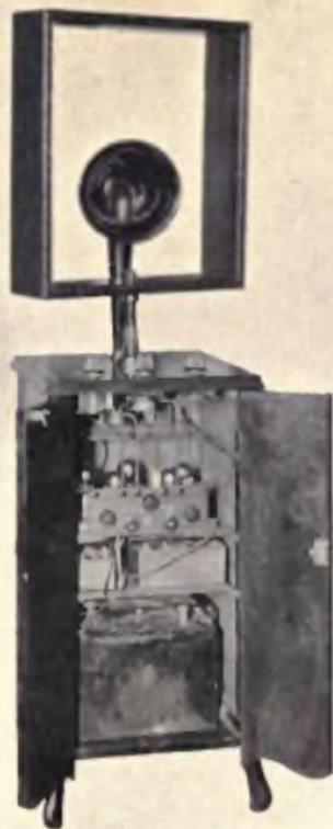
The author's "Radiotrol." This machine was built late in 1921, and is the first radio machine of its class to take on the appearance of a piece of furniture. The Radiotrol, now used in the author's home employs neither antenna nor ground, the reception being made by the loop shown in the engraving. The music, as well as entertainment, from WJZ, Newark, N. J., although twelve miles distant, comes in so loud that the sounds can be heard all over the apartment.
