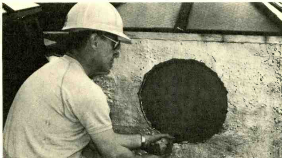
Use a circular rasp to smooth down any rough edges. Make certain you have taken away enough previously that this part of the job isn't harder for you than it should be! The rasp will take care of the final touch, just make sure you get the proper rasp.
