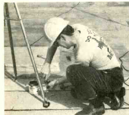
Drive home the lag screws by hand only after all three are most of the way in.
