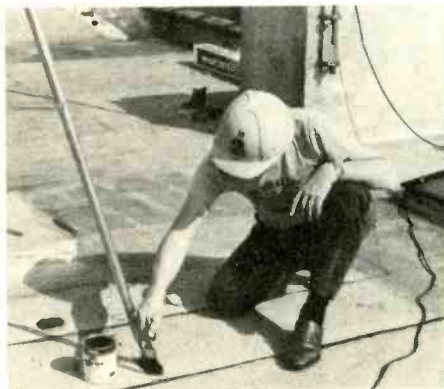
Put roofing compound over the tightened screws to keep them secure and leakproof.
