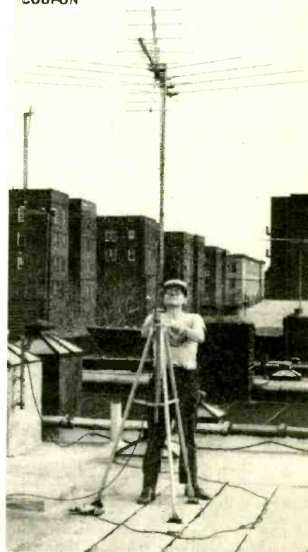
Aim the antenna at the TV transmission tower. Follow the directions in the text.
