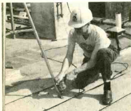
Drill pilot holes for the lag screws and make sure the tower is straight and steady.
