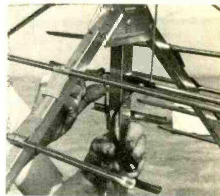
For best results use 75-ohm coaxial cable and an impedance-matching transformer.
