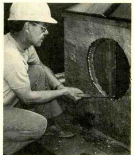
When we came to an obstructing stud, we used a keyhole saw to remove it, but you could use just about any small saw.
