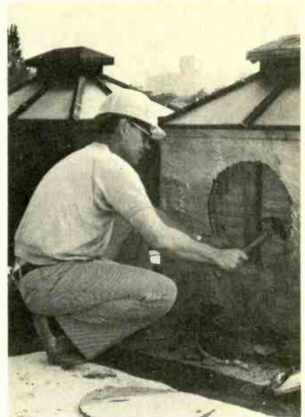
A stud and interior plaster had to be removed. We hammered away splinters and used an old drill bit to do the remainder.
