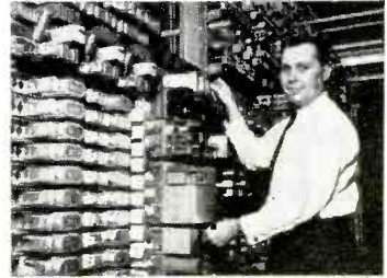
Glenn Horning, Local Equipment Supervisor, Western Reserve Telephone Company.
