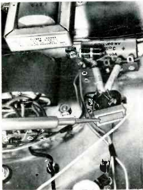
Pointer shows filter resistor to be removed and replaced with filter choke mounted to side of chassis.
