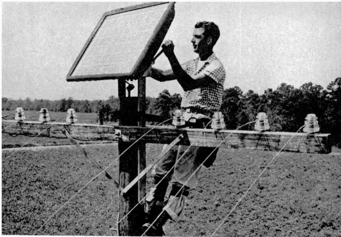
Actual installation of Bell solar battery atop telephone pole near Americus, Georgia. It is being adjusted to best catch sun's rays. The grid of wires, hazily seen along top edge, is lightning discharger.
