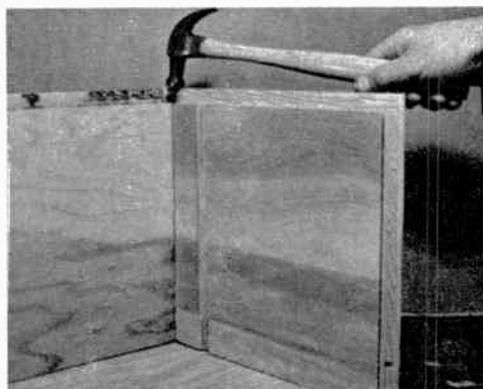
5. With beveled edges of bottom and end panels hand-held, a special clamp nail is driven part—not all the way—into facing slots in bevels.
