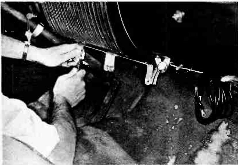
U-shaped brackets for receiver and transmitter cases are being bolted to underhanging lip of dash above transmission hump. Most cars have holes provided there for attaching accessories. Coiled lead will run between battery-generator circuit, receiver, transmitter.
