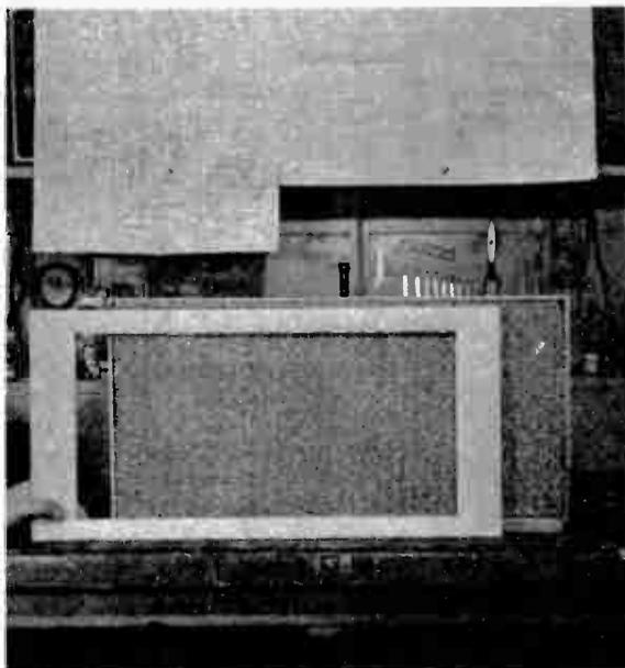
15. The front trim or frame of the SS-1 hi-fi speaker system is supplied completely assembled and it is designed to fit over the entire box-front.
