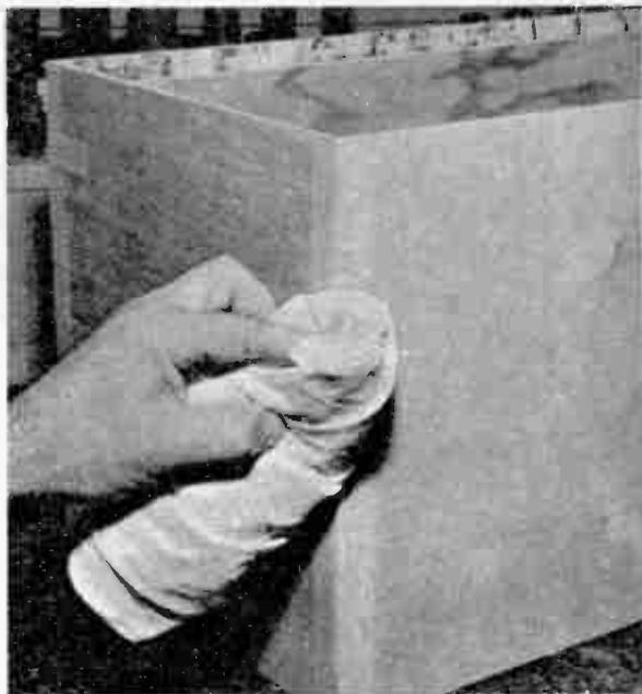
8. Excess glue, squeezed out of joints, is wiped away quickly before it can spread to uncovered surfaces. Allow 15 minutes now for glue to set.
