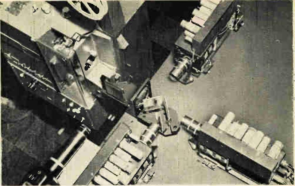
RCA 3-V camera televises color film through a light-splitting optical system that uses Vidicon tubes. Each Vidicon chassis filters its own color portion of original image
