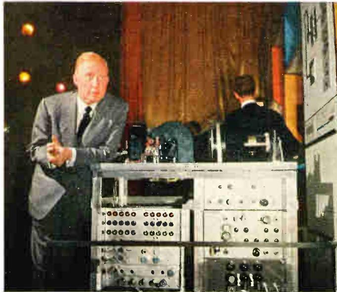
↓ In CBS system, camera sees through a rapidly rotating color wheel. Signals from the camera are in a red-green-blue sequence. After passing through control room, signals go to Chromacoder which converts them into three simultaneous signals for transmission. On the air, signals of CBS and RCA systems are identical
