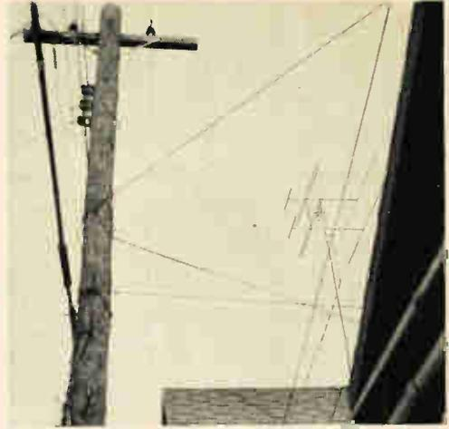
Do not install antenna on damaged chimney and do allow sufficient clearance of power lines
