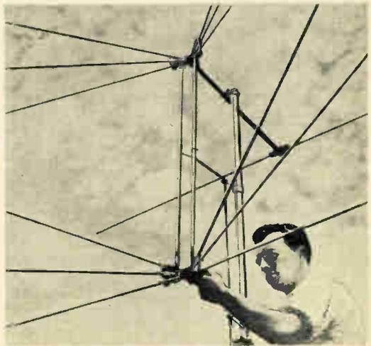
with the desired station. To prevent this, a reflector is added to the antenna. A reflector is an additional element about 5 percent longer than the antenna itself and spaced one quarter of a wavelength behind the antenna. Two advantages come with the use of a reflector: (1) it stops signals from the rear and (2) it tends to add what it receives of the desired signal to the antenna so that it increases the gain.
