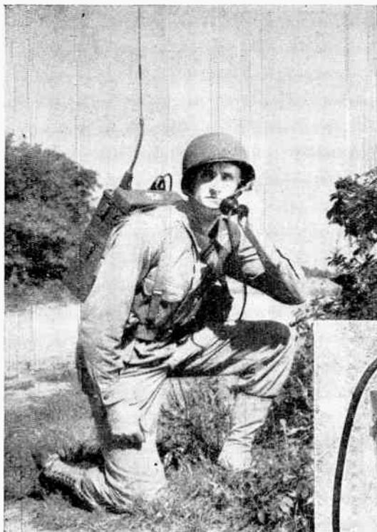
**F.M. WALKIE-TALKIES** developed by the U. S. Army Signal Corps triple the range of the Army's older man-packed radios and have the clarity of tone and static-free transmission and reception associated with frequency modulation. Improved superheterodyne operation facilitates use of two or more sets on the same frequency for intercommunication, while miniature tubes add to compactness and increase battery life.
