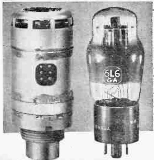
Methods developed to build an entire radio transmitter-receiver into the deadly proximity fuse, here compared in size to a standard radio tube, are used in printing radio circuits for commercial purposes.
