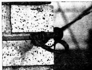
... Leave loops or coils like this in the lead-in near insulators.
