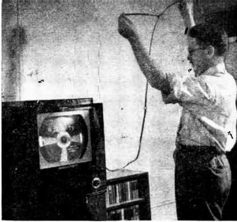
This one-channel antenna may actually surpass a roof antenna. Turn it to face the station.
