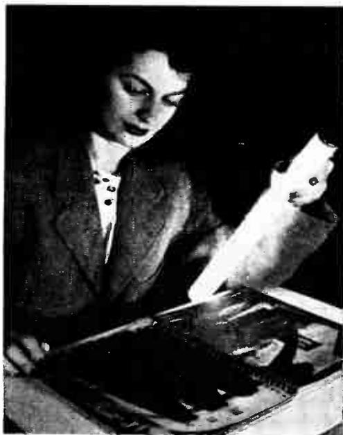
Is this the lighting of the future? The young lady's reading light consists of a fluorescent tube without wired connections. The Tesla coil that powers the tube is located in another room, but plain walls are no obstacle to its energy.
