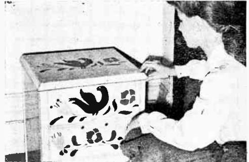
With the old cabinet as a base, construction is held to a minimum. A new and larger loudspeaker is housed in what once was the record compartment.
