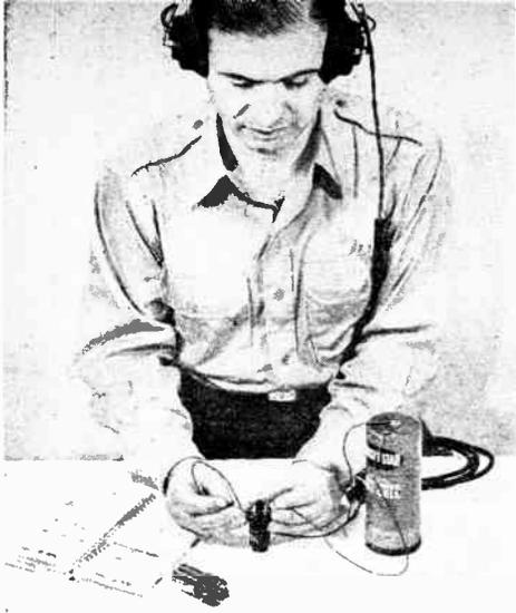
**Heater testing** can be done with any earphones and dry cell. If you hear a loud click when you touch correct base pins (consult a tube chart or the circuit diagram), the filament inside is okay. Otherwise, tube is burned out.
