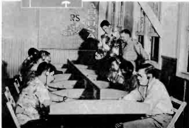
Aspiring amateur radio operators will want these locations sooner or later. Here would-be hams practice code under Signal Corps supervision.
