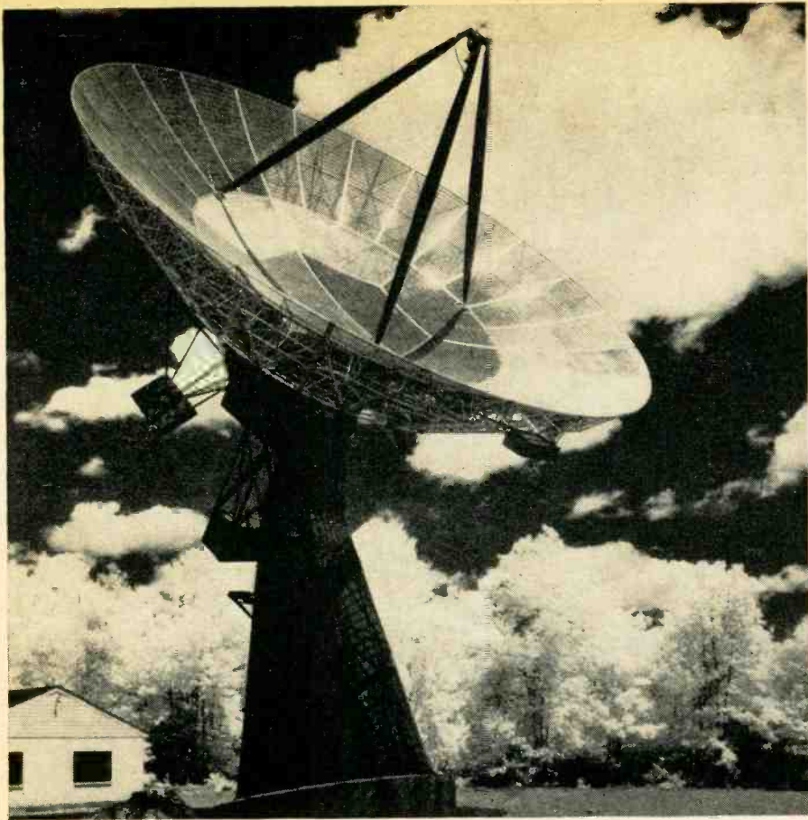
Offset tower supports Harvard University's giant 60-foot radio telescope. Box-like objects hanging from rim of the reflector dish are cement block balancing weights.
