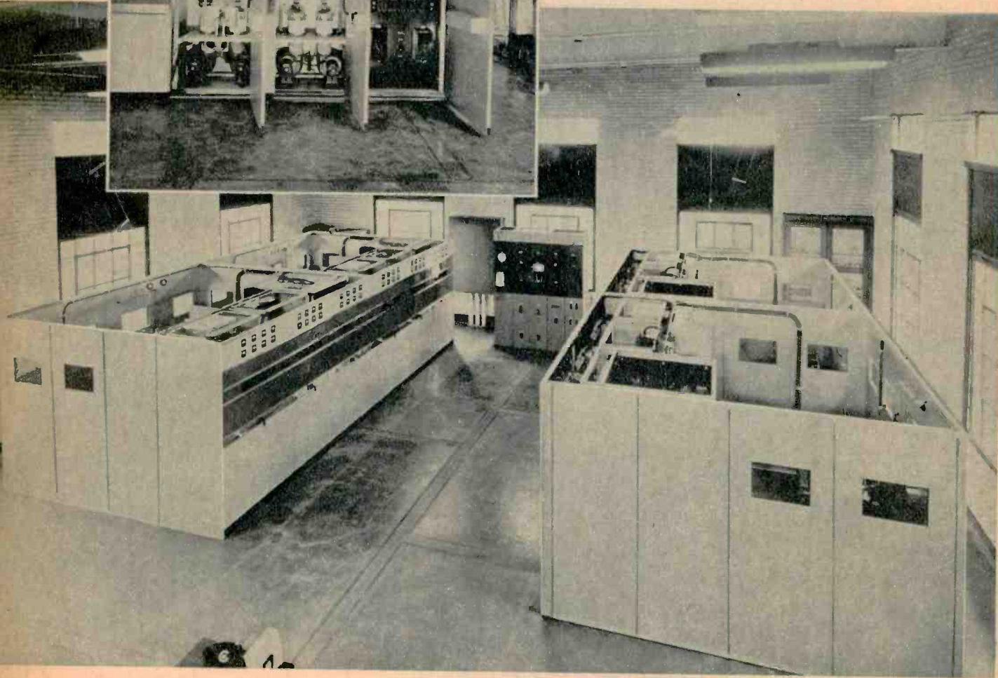
Interior of station WWV, below, shows its four high-power short-wave transmitters that broadcast standard radio frequencies, standard time, etc. Inside of transmitter, inset, shows, left to right, radio-frequency section, audio section, power control panel. Note the motor-fan blowers below two sections, needed since equipment runs 24 hours per day.
