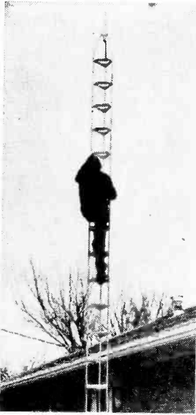
Make sure concrete has cured completely before attempting to climb or work on mast. Poorly set concrete will loosen and crumble.
