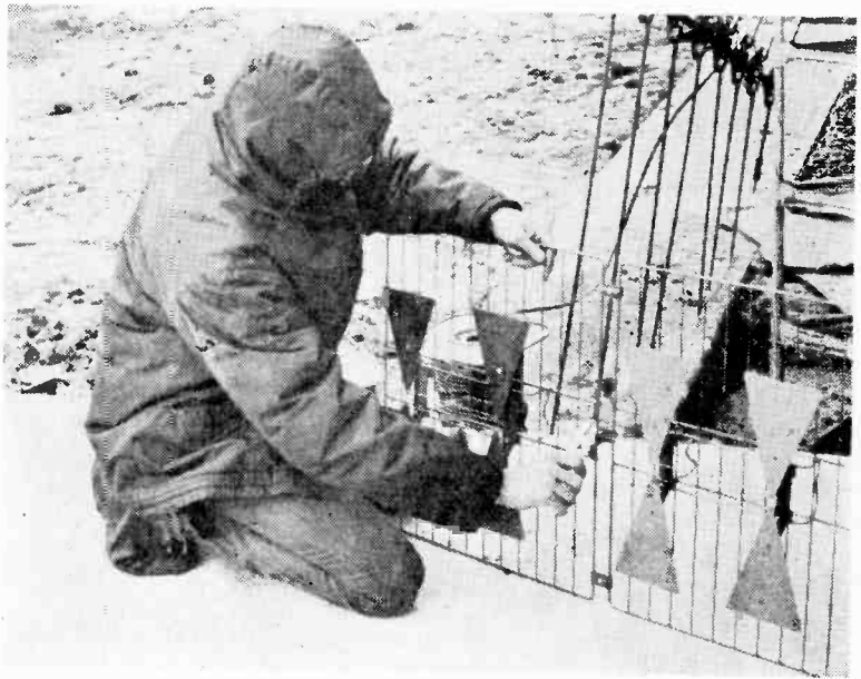
Concrete must be firmly set before you start adding the other sections to the section set in the concrete base.
