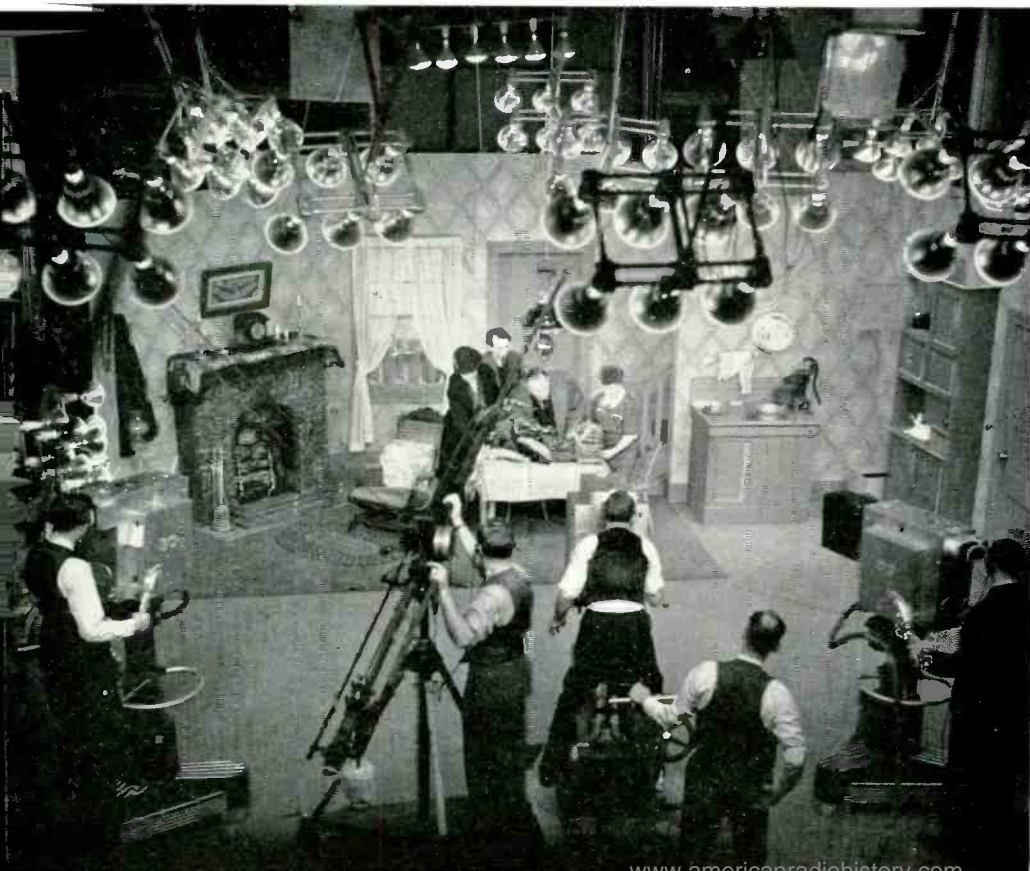
FIG. 2 (at left). A progressive step was the installation of clusters of lights providing greater flexibility.
