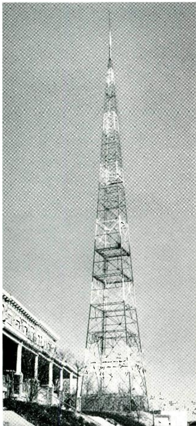
FIG. 3. Self-supporting tower of WBAL-TV, Baltimore, Md. Note the small amount of land area involved and the proximity of tower to residential area.
