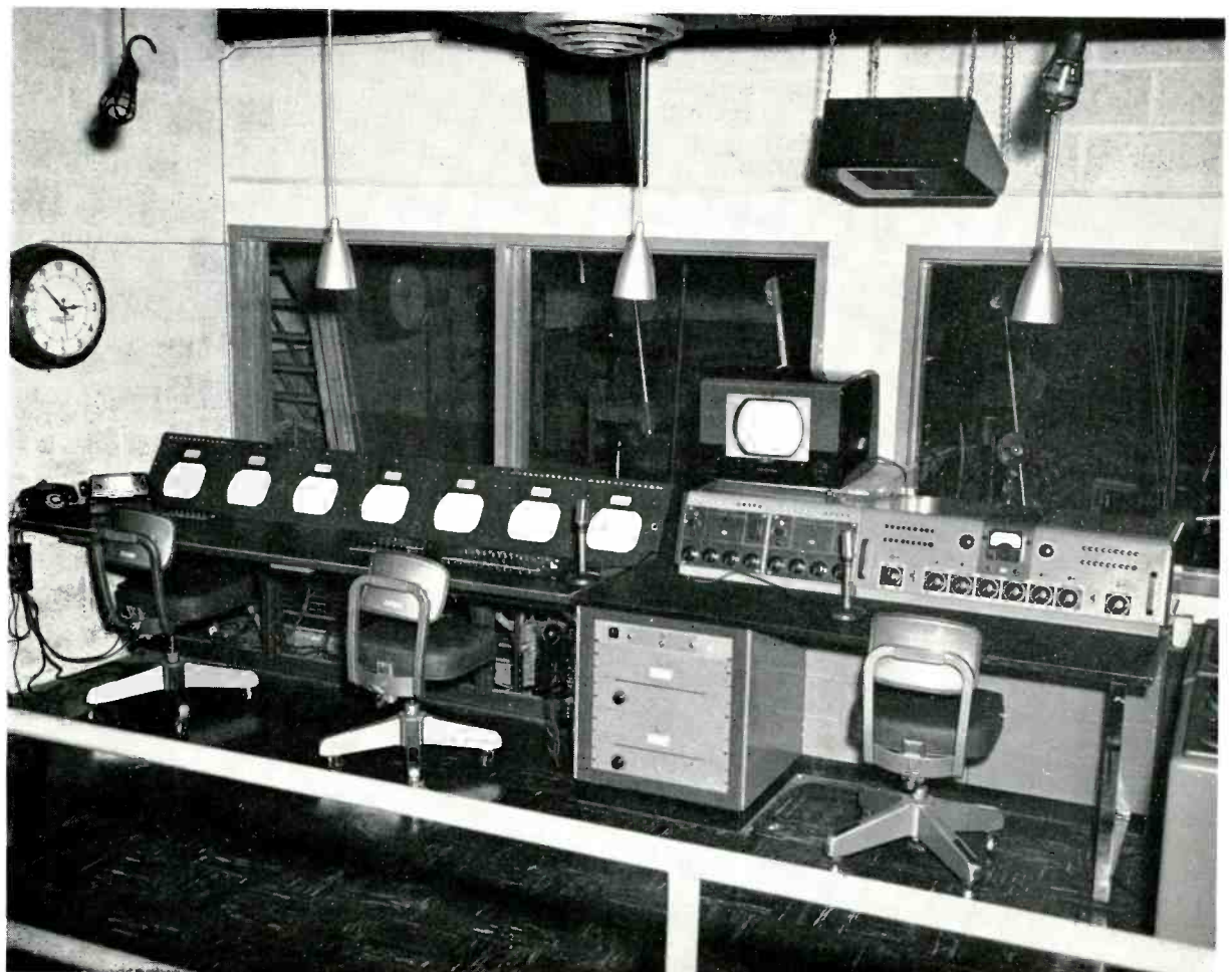
FIG. 11. View of Control Room "A" showing the WOR-TV Program Director's Console at left and the Audio Console at right.
