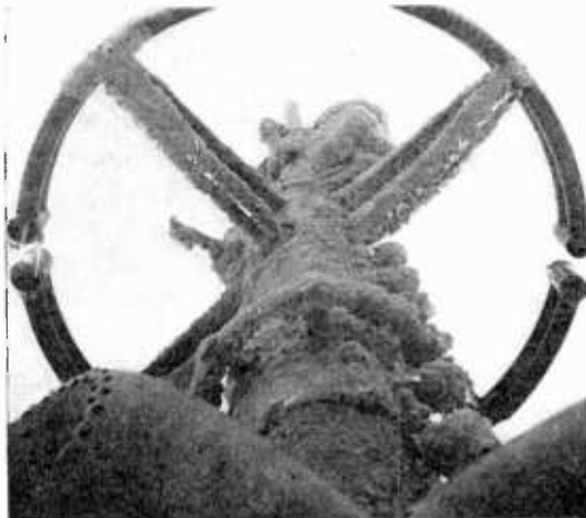
Fig. 21—Ice formation on antenna at Empire State Building. Note the effect from the application of heat to the radiators.
