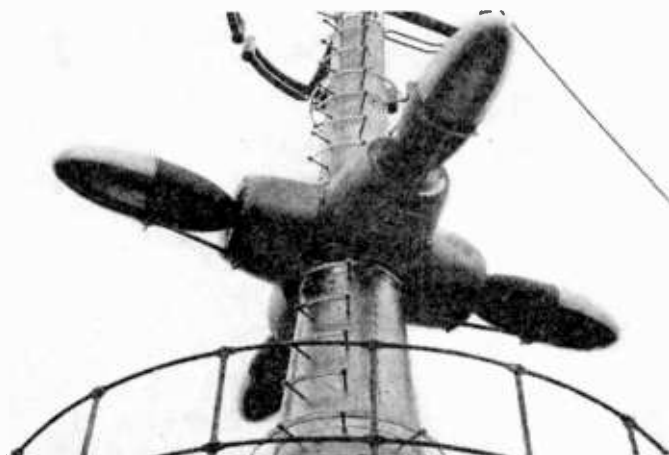
Fig. 12—Empire State Building vision turnstile radiator system.
