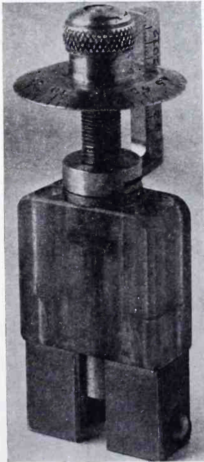
Fig. 10—Balanced condenser for the measurement of resistance by the reactance-variation method.
