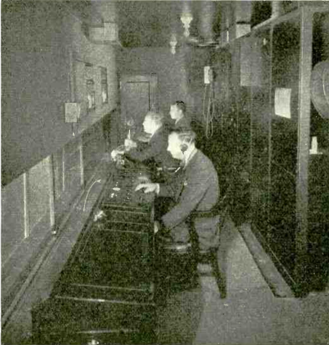
Fig. 4—Television studio control room
