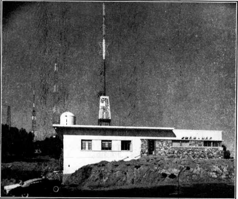
Fig. 21.20. NBC Hollywood Transmitter on Mt. Wilson.
