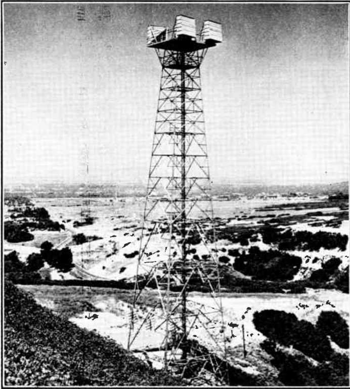
Fig. 21.33. Steel Repeater Tower with Equipment Housed at Base. (Courtesy of American Telephone and Telegraph Co.)
