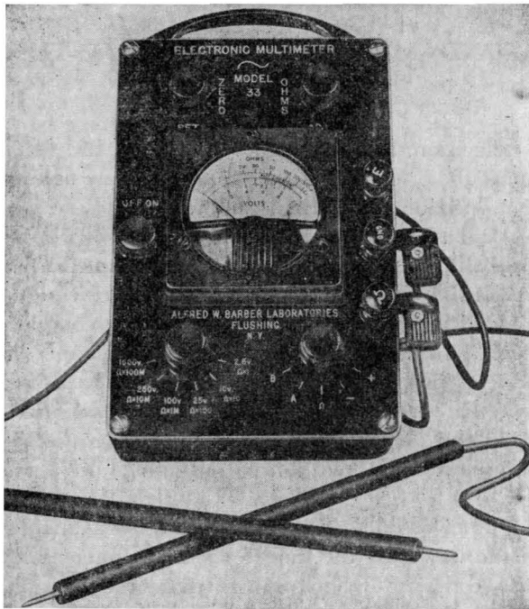
Fig. 1-1. A pocket-size vacuum-tube voltmeter for general purpose use.
