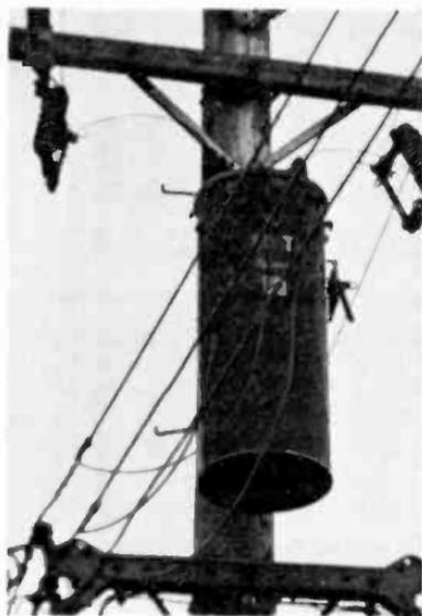
**Fig. 1-3. A typical "pole" transformer, used by the power company to reduce 2400 volts to the 240-volt and 120-volt service brought into your home.**
