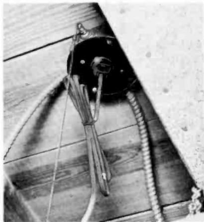
one end around one of the wood screws supporting one box, and loop the other end under a wood screw holding the other adjacent box, running the wire through knock-out holes facing each other on the two boxes. Fig. I-2 shows the wiring of the front outlets. Note the ground wires connected under the wood screws in each of the boxes. This is done the same way that you tied the two right-hand boxes together for grounding.
