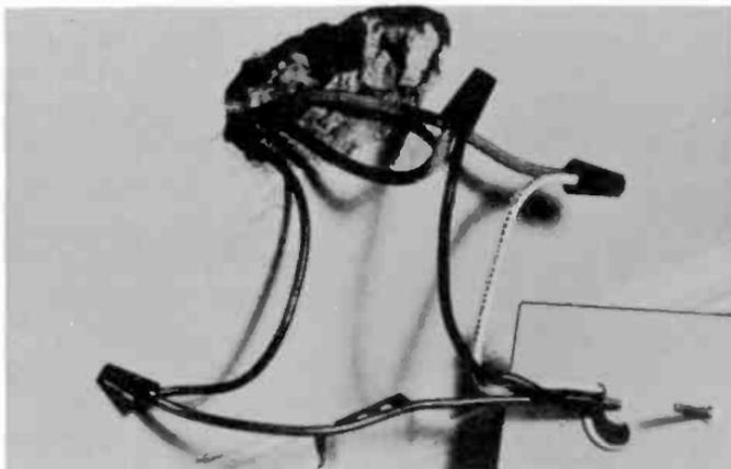
Fig. III-6. A third wire is fastened to the outlet box for grounding. Splice the wires to the "feed-in" cables with wire-nuts.
