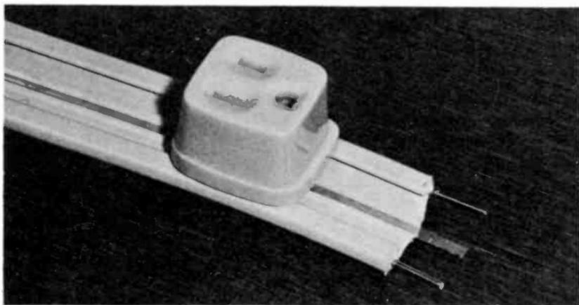
Fig. III-3. Detail of "Electrostrip" surface-wiring cable. Center ribbon is "ground" strip. Outlet twists into grooves and contacts current-carrying wires and ground strip.
