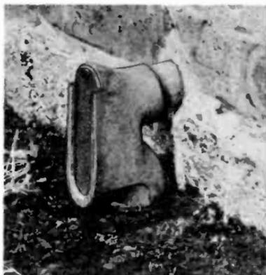
Dig a ditch at least 18 inches deep between the two conduit sections going into the ground, between the house and the garage. The minimum depth required by electrical codes is usually 18 inches. It must be below the frost line and deep enough so that gardening tools will never damage the cable buried in the ditch. It is usually best to follow along an installed fence. You are less likely to dig any deep holes along the fence in the future, and it identifies the location of the cable.
