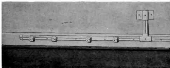
**Fig. III-7.** The finished surface wiring installations. Additional outlets are easy to add; they snap into place anywhere along the cable strip.
