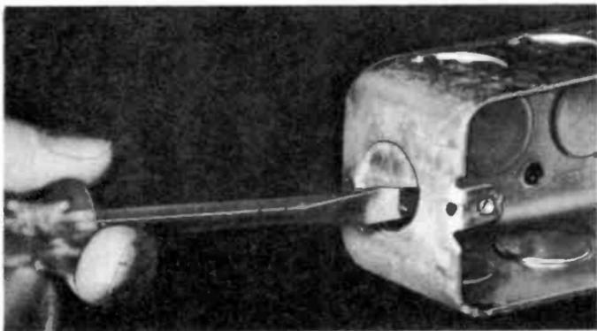
(A) A light tap on a screwdriver pushes the knockout part way out.
