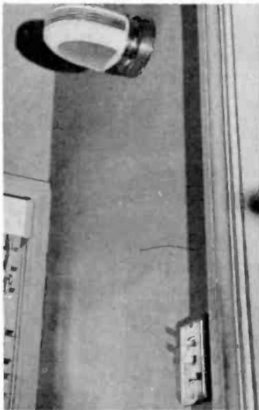
**Fig. IV-2. A back-hall single-light switch was changed to three switches: one for the original hall light; one for the outside floodlight; and a three-way switch for the garage.**
