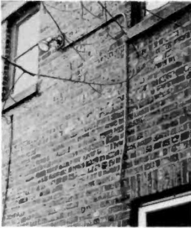
**Fig. IV-1. It is important that wiring to an outside light be fully weatherproof. The use of thin-wall conduit to carry the wires is a must.**
