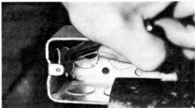
(B) Slug is then removed with pliers.
