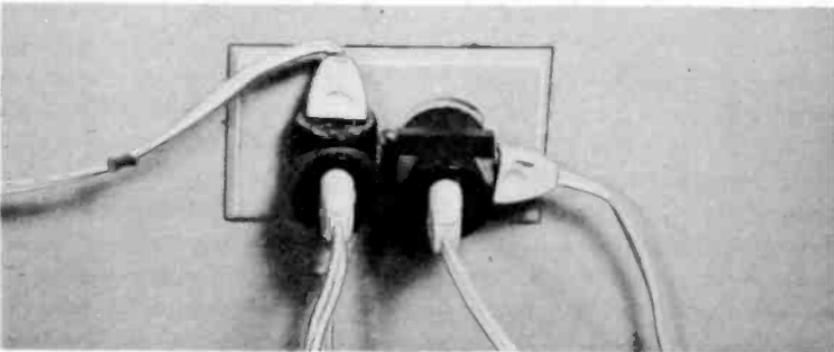
Fig. III-1. A duplex outlet trying to handle five appliances through the use of cube taps. It is hazardous and should be replaced with more outlets.
