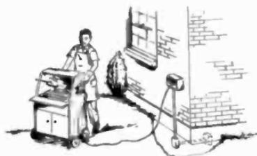
If you have come through brick or concrete for your conduit, be sure to patch up the broken spots afterwards, to keep rain from coming through. In the case of wood, fill in any crevices with plastic wood and, when dry, paint to match the siding.
