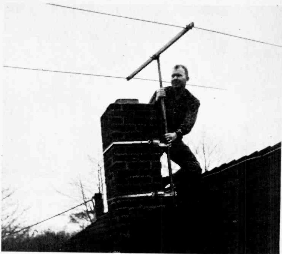
Fig. 56—Often the source of radio frequency interference can be "tuned out" by orientation of the antenna.
