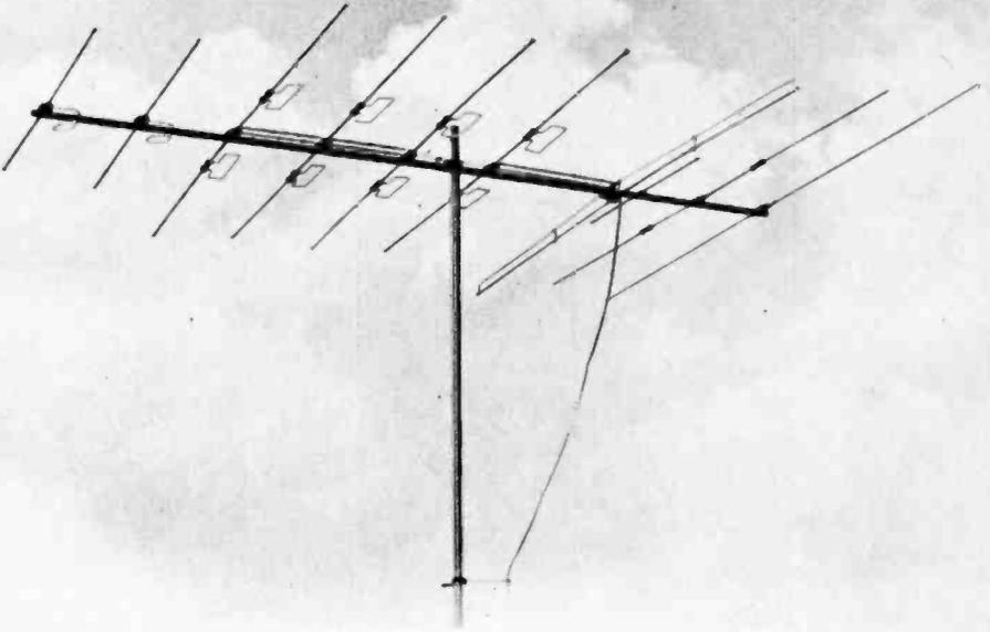
Fig. 45—The element to which the lead-in is connected is called the "driven element." Between it and the TV station are directors, while behind it is the reflector.
