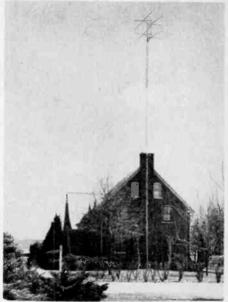
Fig. 52—Typical fringe area installation with 2-bay conical and high, guyed tower.
