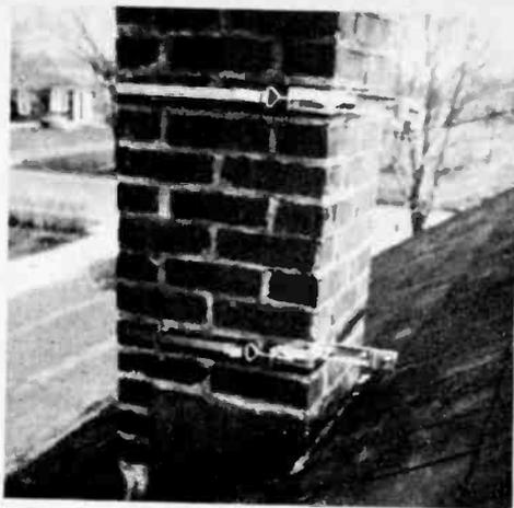
Fig. 49—The chimney mount wraps around chimney, requires no screws to be put in or holes to be drilled.
