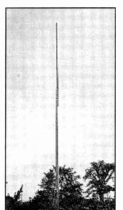
SPLICED TELEPHONE POLES MAKE AN IDEAL MAST FOR EXPERIMENTAL ANTENNAS
