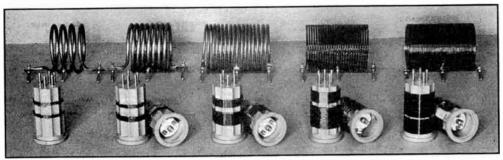
FIG. 938 — A COMPLETE SET OF COILS FOR OPERATION IN FIVE BANDS WITH CRYSTALS GROUND FOR FOUR BANDS
