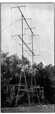
FIG. 1625 - A TYPICAL RIGID MOUNT-FOR THE ULTRA-HIGH FRE-OUENCY DIRECTIVE ARRAY
