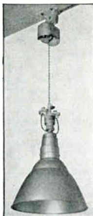
A Typical High Bay Installation, Partially Lowered
