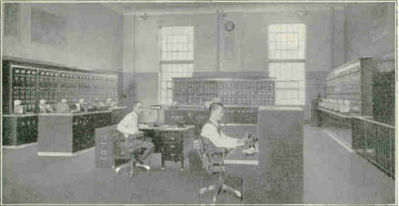
Installation at Cincinnati, Ohio
