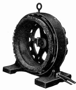
Fig. 331. Primary Member of Westinghouse Induction Motor Completely Wound
