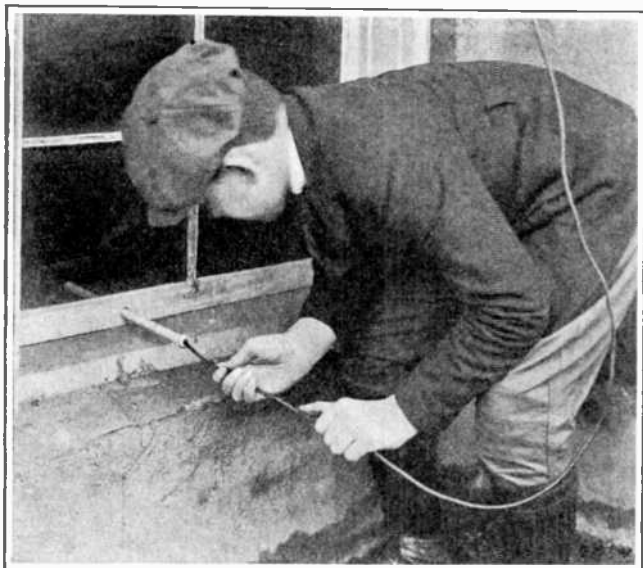
It is best to pass all wires through porcelain tubes when they enter the house, as shown here, even though the wires may be heavily insulated. It is an additional precaution well worth taking.
