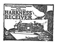
The Harkness Receiver is essentially a Reflex circuit which successfully employs tuned radio frequency amplification without the necessity of using a potentiometer or neutralizing condensers to prevent self-oscillation. Those who are familiar with radio circuits and their operation will readily realize the importance of this achievement in radio frequency amplification and will be astonished with the remarkable sensitiveness and selectivity of this set.
