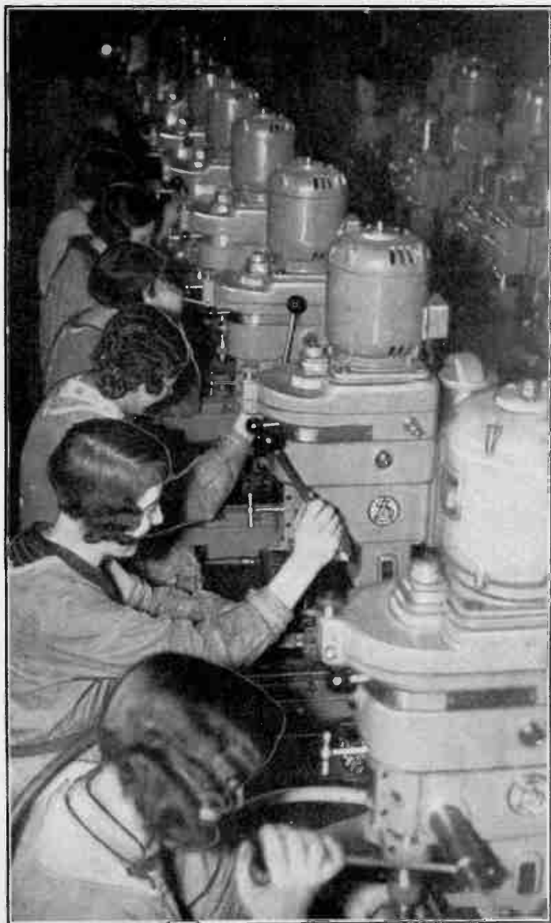
STAMPING OUT PARTS REQUIRED IN VALVE CONSTRUCTION
