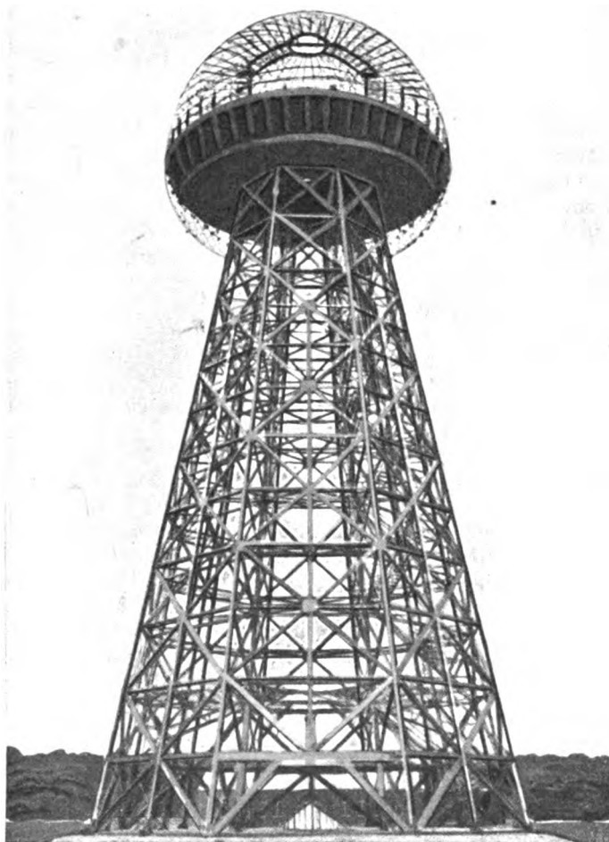
FIG. 125.—MR TESLA'S TRANSMITTING STATION ON LONG ISLAND.
