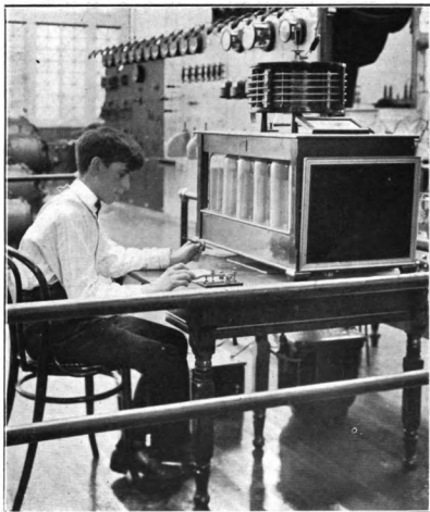
FIG. 86. —Interior of a De Forest Station.
