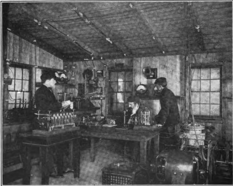
FIGURE 136—National Electric Signaling Company-Fessenden 2 K. W. radiophone transmitter.
