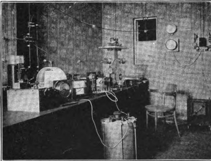
FIGURE 36—Ruhmer's radiophone transmitter.
