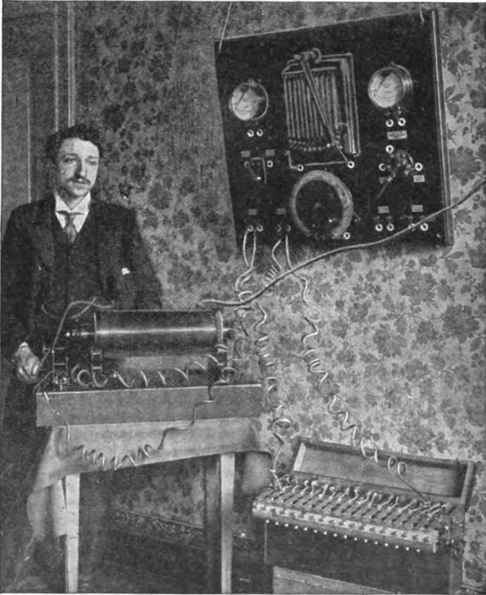
FIG. 172.—GUARINI TRANSMITTER. (First Form.)
