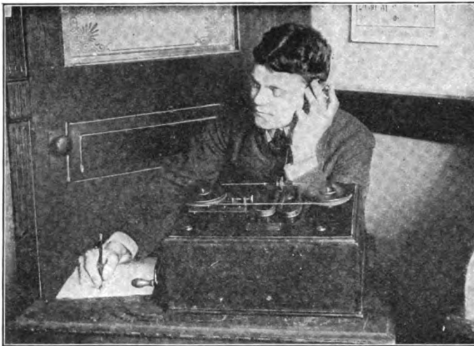
FIG. 157.—MARCONI MAGNETIC DETECTOR.
