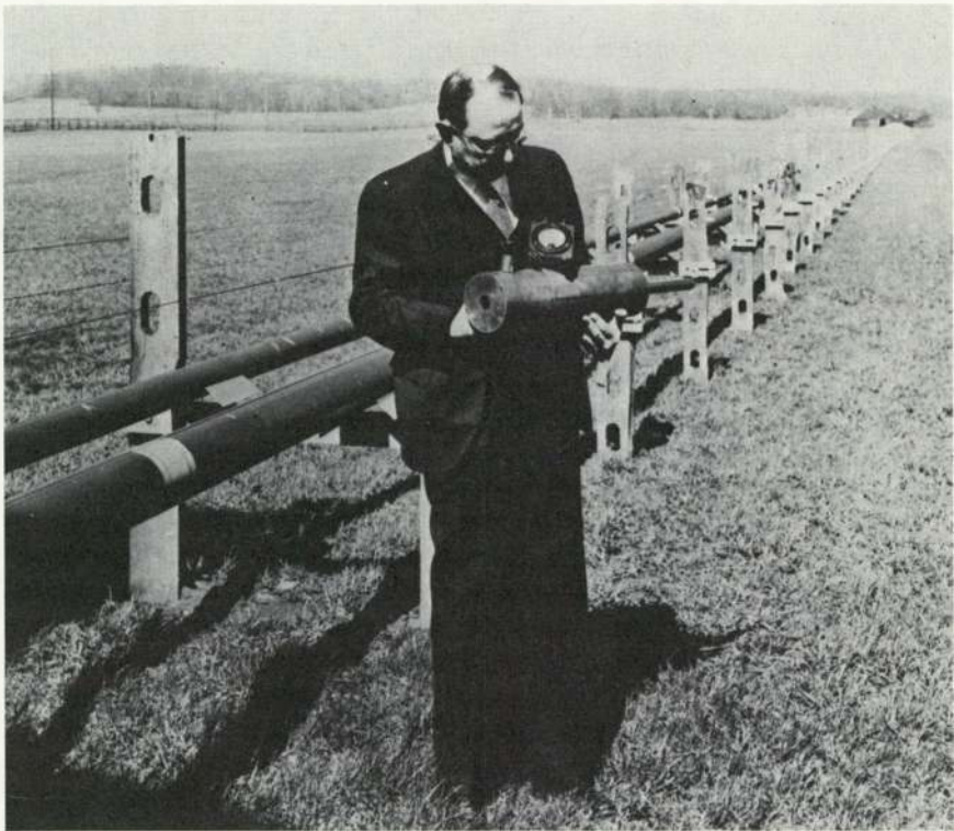
Fig. 6-1. G. C. Southworth in front of a TE_{01} waveguide transmission line built at Holmdel, New Jersey, in 1935. Southworth holds one of the resonant chambers used for tests of waveguide transmission.
