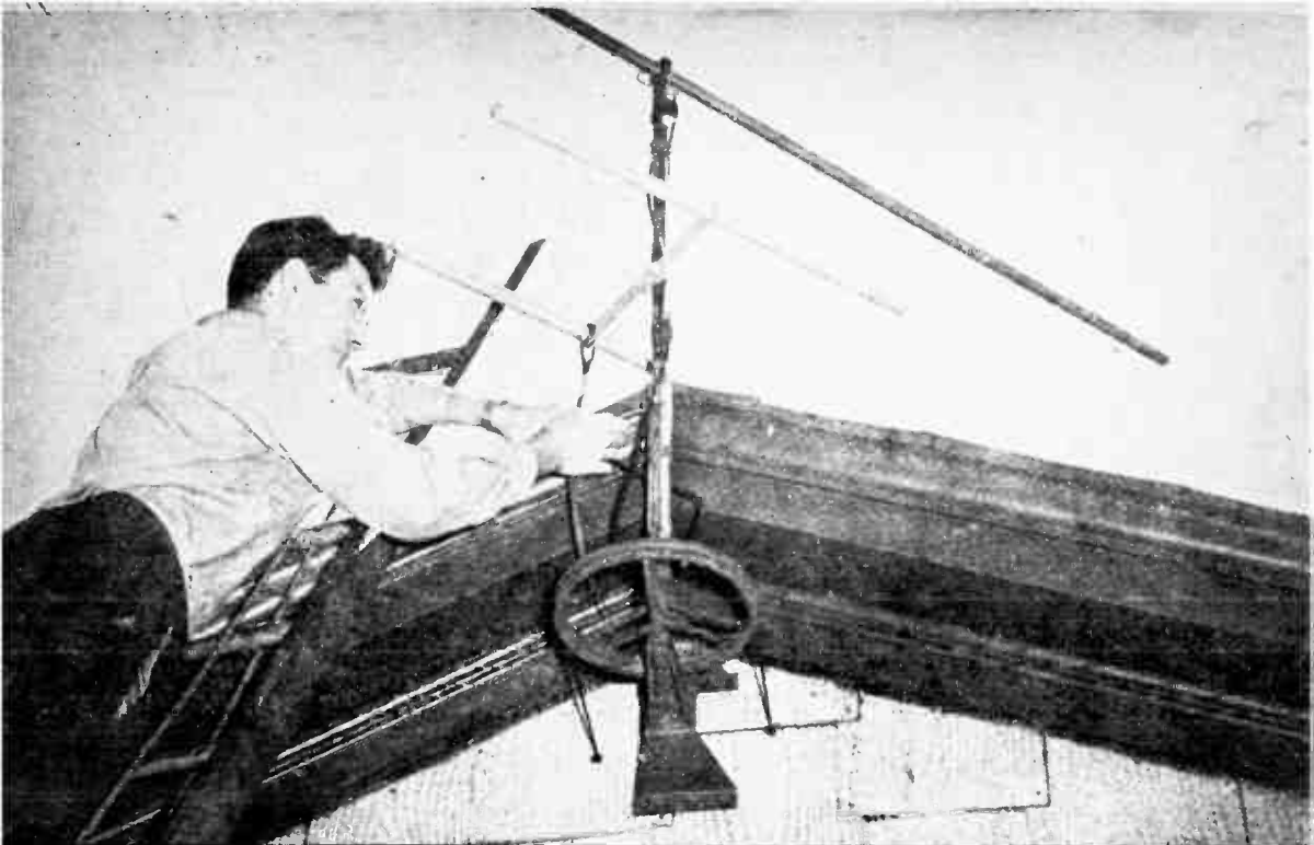
Placing the outside pulley near the roof peak allows the mast to be cut to a short stub.
