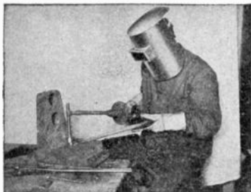
FIGS. 4,499 and 4,500.—C and C electric arc welding apparatus. Fig. 4,499, operator with one type of head shield and combination electrode holder for both metallic and graphite electrodes. Fig. 4,500, graphite electrode holder and hand shield.
