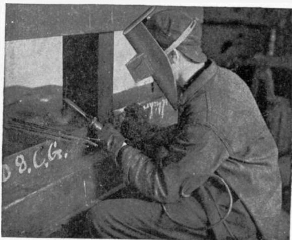
Fig. 4,501.—Operator using C and C electric arc welding metallic electrode. The electrode itself is melted and supplies the extra metal necessary for welding or building up.
