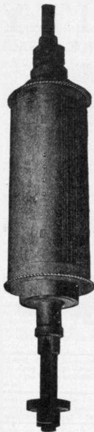
FIG. 1,583.—Westinghouse two pole parallel slot turbine alternator field.
