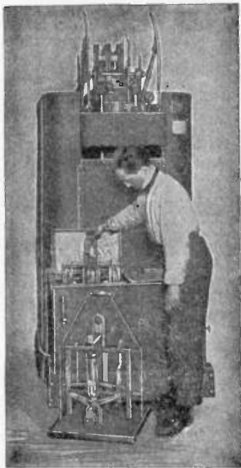
FIG. 2,119.—General Electric series mercury arc rectifier outfit; view showing method of replacing a tube. The illustration also shows tube carrier and drip tray.
