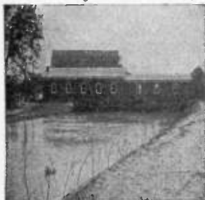
FIGS. 2,769 and 2,770. —Exterior and interior of hydro-electric plant at Harrisburg, Va. It is located on the south fork of the Shenandoah River, twelve and one-half miles distant. A dam 720 feet long and 15 feet high was built on a limestone ledge running across the river; which with a fall of 5 feet from the dam to the power house, a quarter of a mile distant, secured an effective head pressure of 20 feet. The power house, comprising the generator room and the wheel room, also the machinery room, are here shown. The wheel room, which is 20 × 40 feet, extends across the head race, and rests upon solid concrete walls, forming the sides and ends of the wheel pits. The end wall is 6 feet thick at the bottom, and 4½ feet at the top. It has three arched openings, each 8 feet wide and 9 feet high, through which the water escapes after leaving the turbines. The intake is protected by a wrought iron rack 40 feet long. The power is obtained by three 50 inch vertical shaft Samson turbines, with a 20 inch Samson for an exciter. The three large turbines have a rating of 1,350 horse power; and are connected to the main horizontal line shaft by bevel mortise gears 7 feet diameter and 15 inches face. The couplings on the main shaft have 48 inch friction clutch hubs, permitting either or each turbine being operated, or shut down independently of the others. The main shaft is 85 feet long and 6 inches diameter; making 280 revolutions. This shaft carries two pulleys 70 inches diameter and 38 inches face for driving the generators. The accompanying illustration shows the harness work, gears, pulleys, etc., furnished with the turbines. The 20 inch horizontal shaft Samson turbine of 72 horse power is direct connected to an exciter generator of 20 kw., running 700 rev. per min. The two large generators are driven 450 revolutions per minute by belts producing a three phase current of 60 cycles of 11,500 volts for the twelve and one-half miles transmission. The line consists of three strands of No. 4 bare copper wire. This current is used for lighting and power purposes, and the plant is of the latest improved design and construction.
