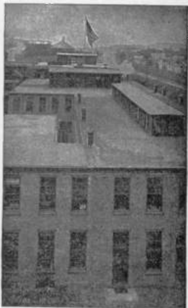
FIGS. 2,739 and 2,740. —Substituting mechanical draught in place of chimney. The relative proportions of a brick chimney, and of the smoke pipe required when mechanical draft is introduced are forcibly shown in the illustrations, which show the works of the B. F. Sturtevant Co., at Jamaica Plain, Mass. The removal of the boilers to a position too far distant from the existing chimney to permit of its longer fulfilling its office, led to the substitution of an induced draft fan and the subsequent removal of the chimney. The present stack or smoke pipe, barely visible in fig. 2,740, extends only 31 feet above the ground, and no trouble is experienced from smoke.
