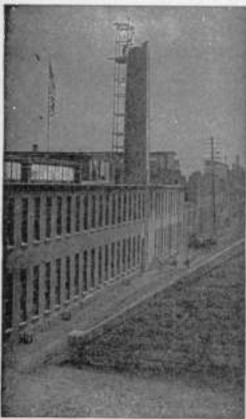
FIGS. 2,739 and 2,740. —Substituting mechanical draught in place of chimney. The relative proportions of a brick chimney, and of the smoke pipe required when mechanical draft is introduced are forcibly shown in the illustrations, which show the works of the B. F. Sturtevant Co., at Jamaica Plain, Mass. The removal of the boilers to a position too far distant from the existing chimney to permit of its longer fulfilling its office, led to the substitution of an induced draft fan and the subsequent removal of the chimney. The present stack or smoke pipe, barely visible in fig. 2,740, extends only 31 feet above the ground, and no trouble is experienced from smoke.
