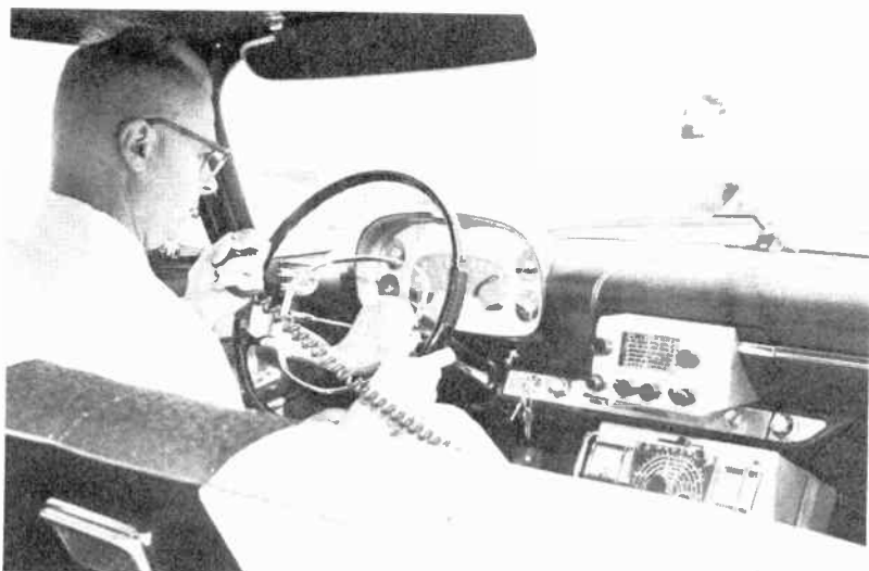
13-3. Separate receiver and transmitter are used in this mobile installation. Part of glove compartment has been sacrificed to make room for the former. In this position it is within reach of operator.
