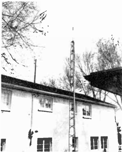
12-5. This self-supporting tower with a top mast section is a five-band vertical antenna that requires little ground space. Overall height is about 50 feet. (Courtesy High-Gain Antenna Products Corporation.)
