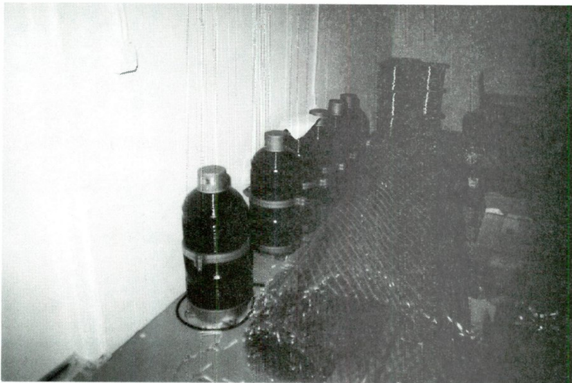
photo 3.3 – Beacon lights, rolls of copper ground mat, and spools of copper wire await installation at a new AM tower construction site.
