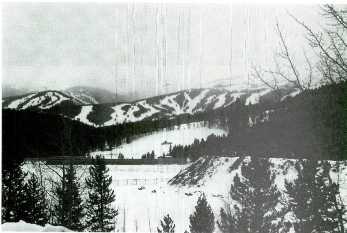
photo 3.4 – The large circular clearing surrounding the antenna tower near the center of this photo is an example of the need to remove obstructions from the antenna field.
