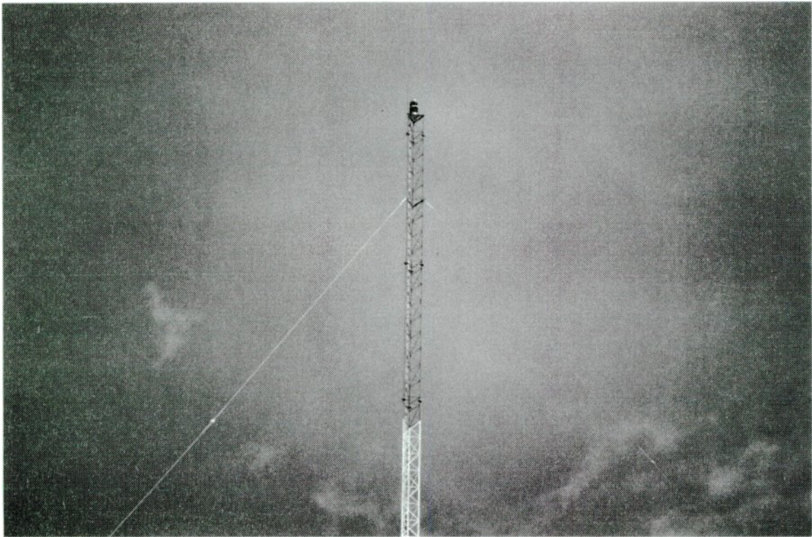
photo 6.14 – Part of the station's ongoing maintenance costs might include the cost of repainting and relamping the towers on a regular basis. One local AM station told the author that they usually pay about $1 per foot of tower height for someone to climb the tower and replace the lights.
