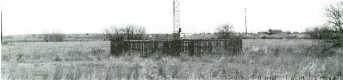
photo 6.5 – Fencing helps to prevent unauthorized persons from getting too close to the electrically energized base of an AM tower.
