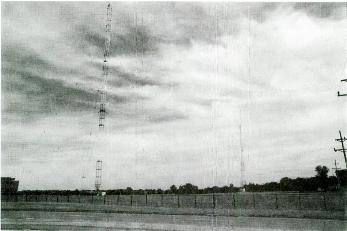
photo 4.16 – The 680 foot guyed main tower (left) and the 250 foot self-supporting auxiliary tower (right) of WBBM/780 in suburban Chicago, IL.
