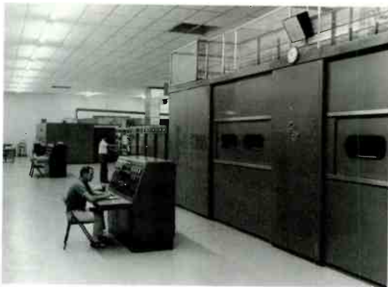
Fig. 1-5 This is Transmitter Hall at Trans-World Radio in the sunny Netherlands Antilles. TWR's huge 500kW (800kHz) AM broadcast transmitter is shown being monitored from the foreground console. A 260kW shortwave broadcast transmitter is being adjusted in the background. (TWR photo)
