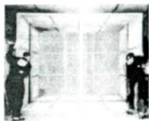
ADDING FILLER SECTIONS Additional sections are added as required to enlarge room to proper length.
