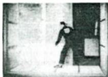
STARTING SECTION Floor panel is placed in position. Two wall panels are positioned to form a corner. Additional wall panels are added to complete section.
