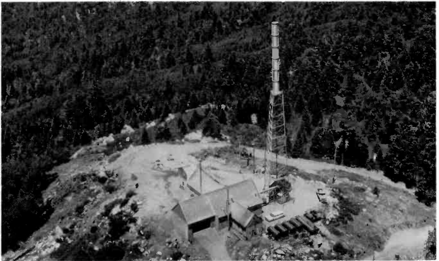
Fig. 2-5. This antenna location is 3697 feet above average terrain at an altitude of 7622 feet above sea level. Used by KERO-TV, Bakersfield, California, the antenna is enclosed in a radome for protection from severe weather. (GE)
