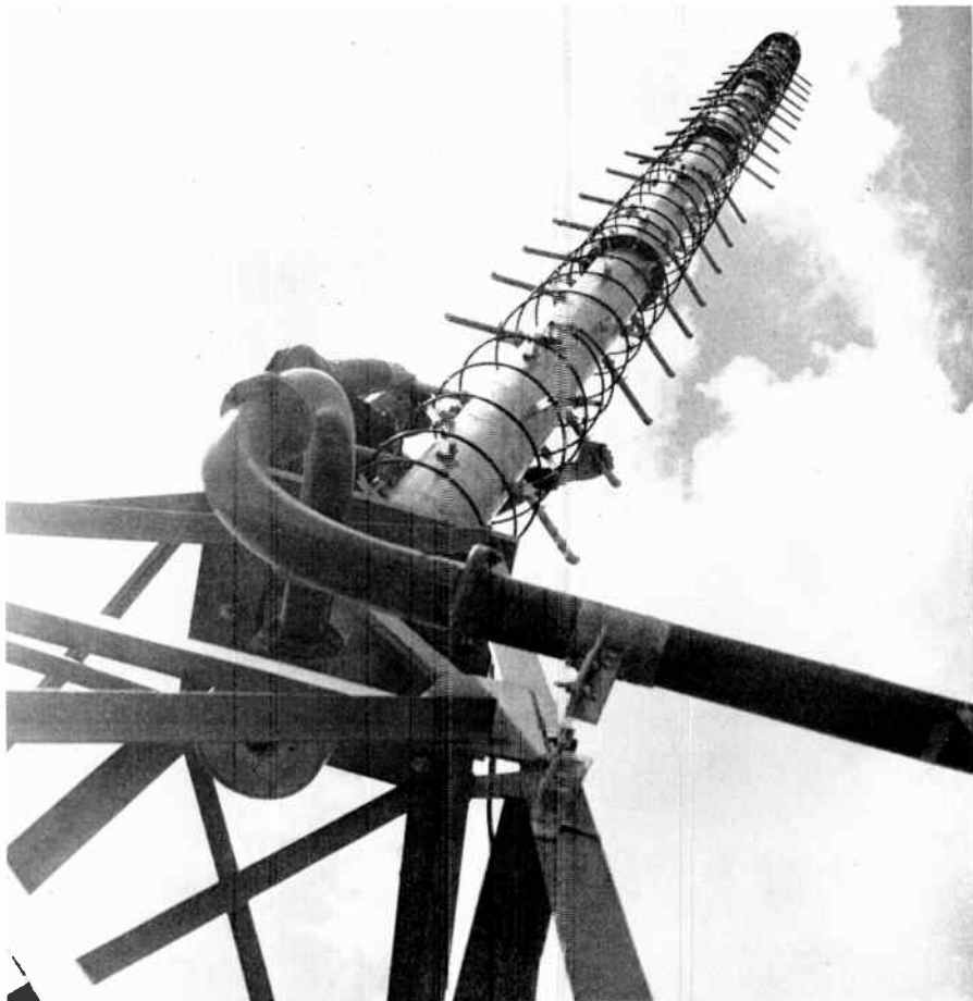
Figure 5.4E. Broadcast television 4-bay UHF high-gain helical transmitting antenna, type TY-24-A, for channels 14 through 19. Courtesy General Electric.
