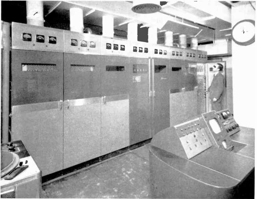
Figure 1.14A. RCA TT-5A transmitter at WENR-TV, Chicago, Courtesy RCA.
