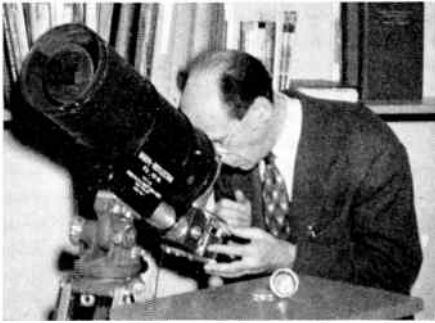
Figure 2.1P. Dr. Frank G. Back, inventor of the Television Zoomar Lens, the Video Balowstar, the 40-inch Reflector and the Video Analyzer, testing a 40-inch Reflector Lens now used extensively for remote pickups of baseball, football, horse racing, soccer, aviation, parades, etc. Courtesy Back Video Corporation.
