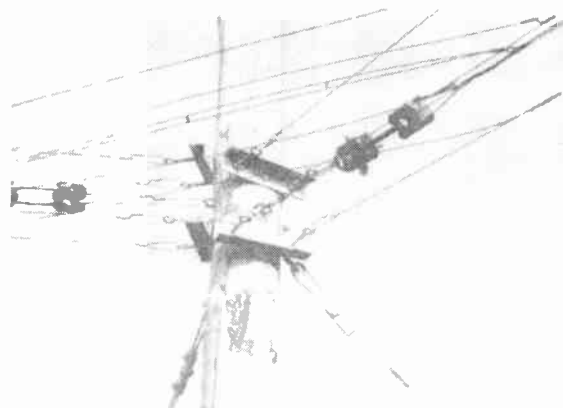
FIG. 4.73. Details of a corner pole for a feeder of the six-wire unbalanced type built on untreated wood pole with steel-angle crossarms. The high-potential pair of wires is insulated by means of double-egg porcelain insulators with steel yokes. Spacers are used between the two inner wires to maintain uniform spacing. (Photograph courtesy of RCA Victor Company, Ltd., Montreal.)
