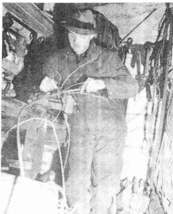
FIG. 3.107. Inside a rigger's hut during a steel-rope splicing operation. Notice typical rigging equipment in background.
