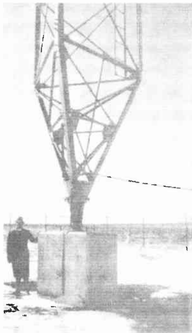
FIG. 2.55. A top-loaded sectionalized guyed vertical radiator and its base detail. Radio Station WMAQ, Chicago, Illinois. (Photograph courtesy of National Broadcasting Company.)
