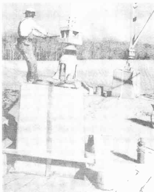
FIG. 2.56. Base of a self-supporting broadcast radiator during construction. Notice tractor and plow tracks in background where ground wires have been plowed into the soil. (Photograph courtesy of National Broadcasting Company.)
