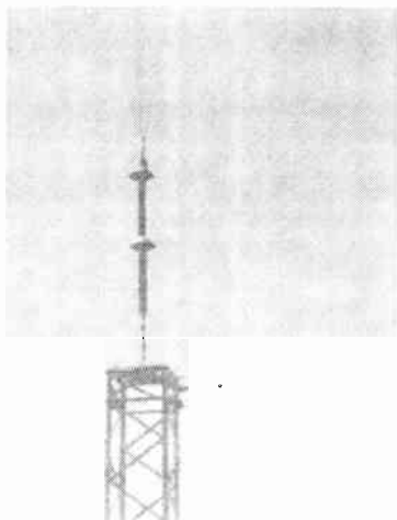
FIG. 1.41. Down-lead insulator and the end of the six-wire unbalanced unmatched feeder for the antenna of Fig. 1.5.
