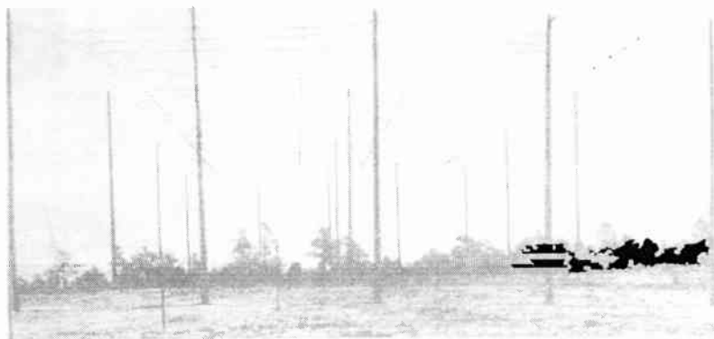
FIG. 3.121. A two-bay fishbone receiving antenna as used at the Riverhead Receiving Station of RCA Communications, Inc.
