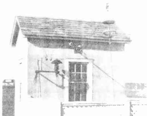
FIG. 1.36. Antenna down-lead and coupling-house-entrance detail as used at medium-power low-frequency stations.
