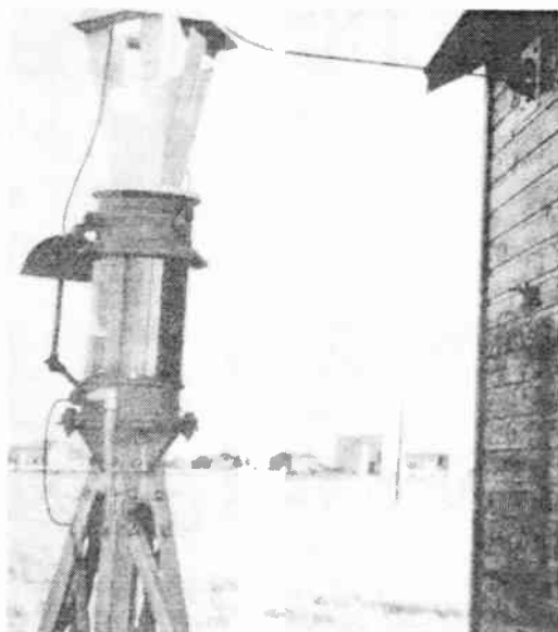
FIG. 2.64. Base insulator of the Austin oil-filled safety-core type with the tower-lighting transformer located inside the base insulator, at Station CKLW. (Photograph courtesy of RCA Victor Company, Ltd., Montreal.)
