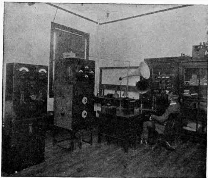
FIG. 79. Interior of broadcasting station showing transmitting apparatus.
